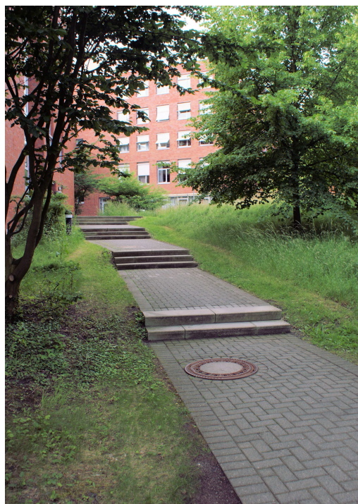
Picture 3. Slopes causing problems for mobility impaired people or wheelchair
