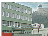
Regional Office SAO Trenčín
